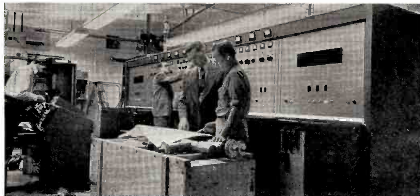
G-E field engineers Stone, Bias and Duncan (l. to r.) work on the installation of the first 12 kw transmitter built by G.E. for WHUM-TV.
